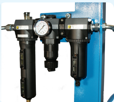
Filter Regulator Lubricator
